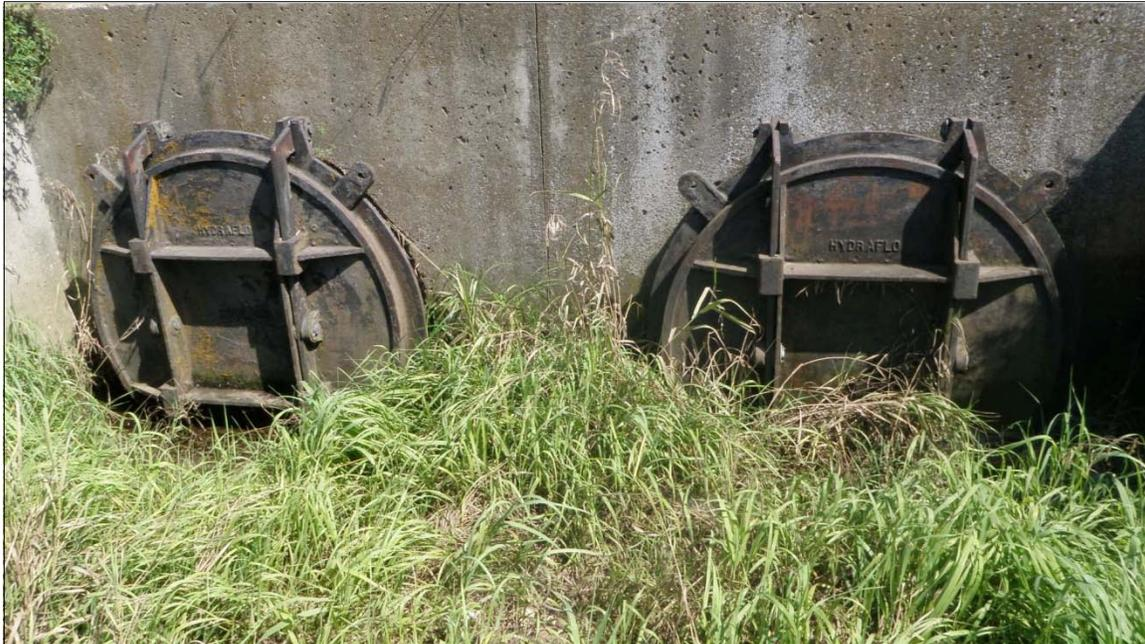
Figure 4. Field drainage outfalls blocked by sediment deposition
