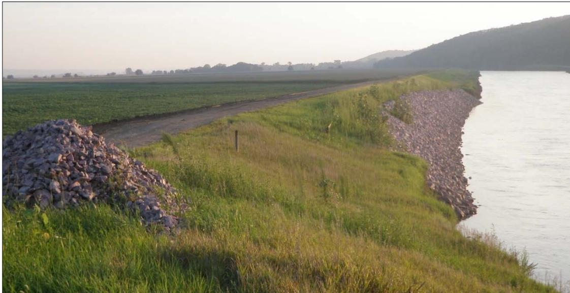
Figure 2. Loss of riverside levee to erosion
