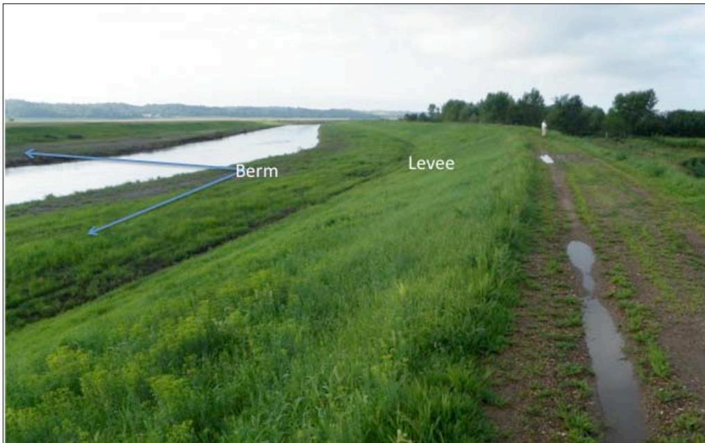
Figure 1 Typical levee section with berms
